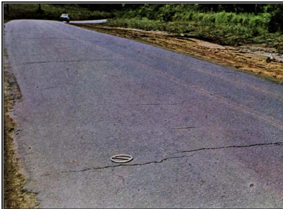
**Figura 3.2:** Trincamento Transversal, DNIT (2003)
