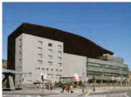
Figura 97 – Euskalduna Convention Centre (Bilbao) Fonte: http://www.operahouseweb.com/wp-content/uploads/2011/11/euskalduna-conference-centre-and-concert-hall.jpg
