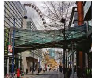
Figura 143 – Ponte sobre a Corporation Street (Manchester)
